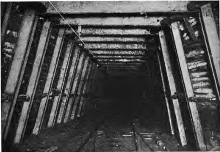
Fig. 6. Steel Framed Gangway, Style A., Summit Branch Mining Co., Williamstown, Pa.
